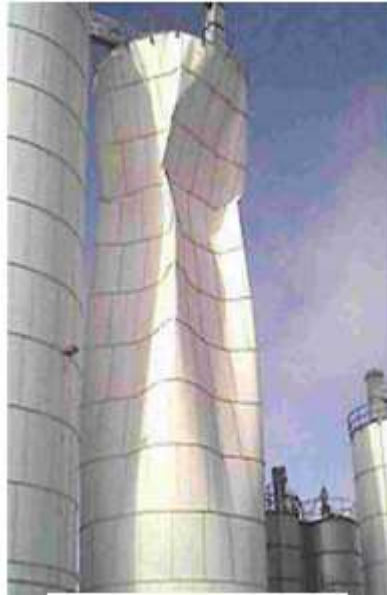
Figure 1: Buckled Silo
